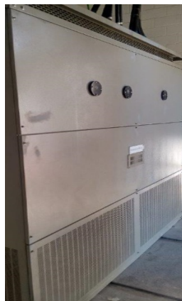
Example of thermographic windows installed in a dry transformer aligned with the internal connections (Images from the JIT Brasil archive).
