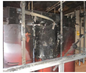
Dry insulation transformers damaged as a result of short circuit – without thermography (Image from JIT Brazil archive).
