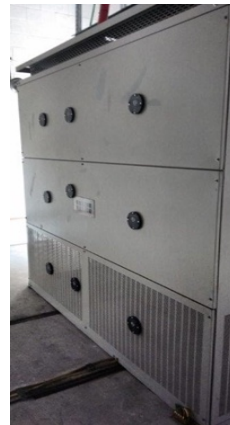
Example of thermographic windows installed in a dry transformer aligned with the internal connections (Images from the JIT Brasil archive).
