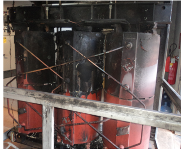
Dry insulation transformers damaged as a result of short circuit – without thermography (Image from JIT Brazil archive).
