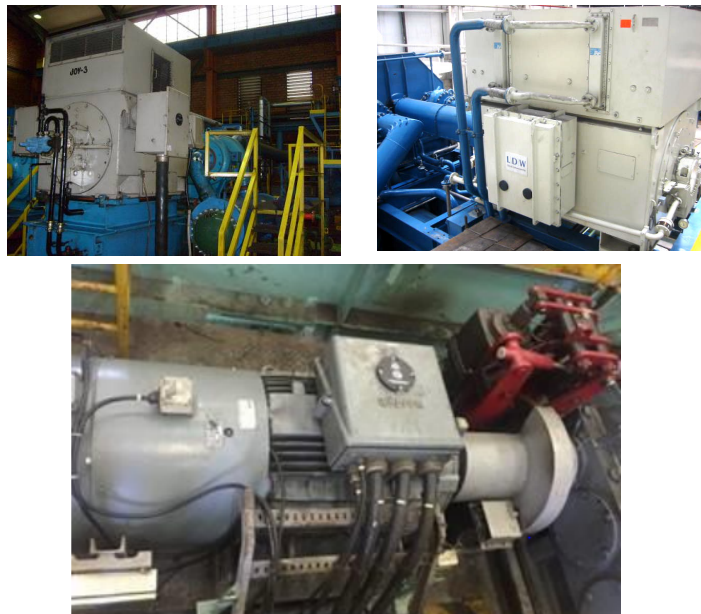
Examples of thermographic window installation in electric motors (images from the JIT Brasil file).
