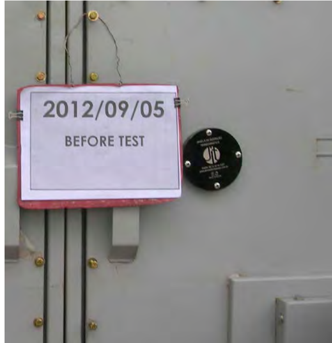
Photo 5 – Before test (InfraPred JIT75)
