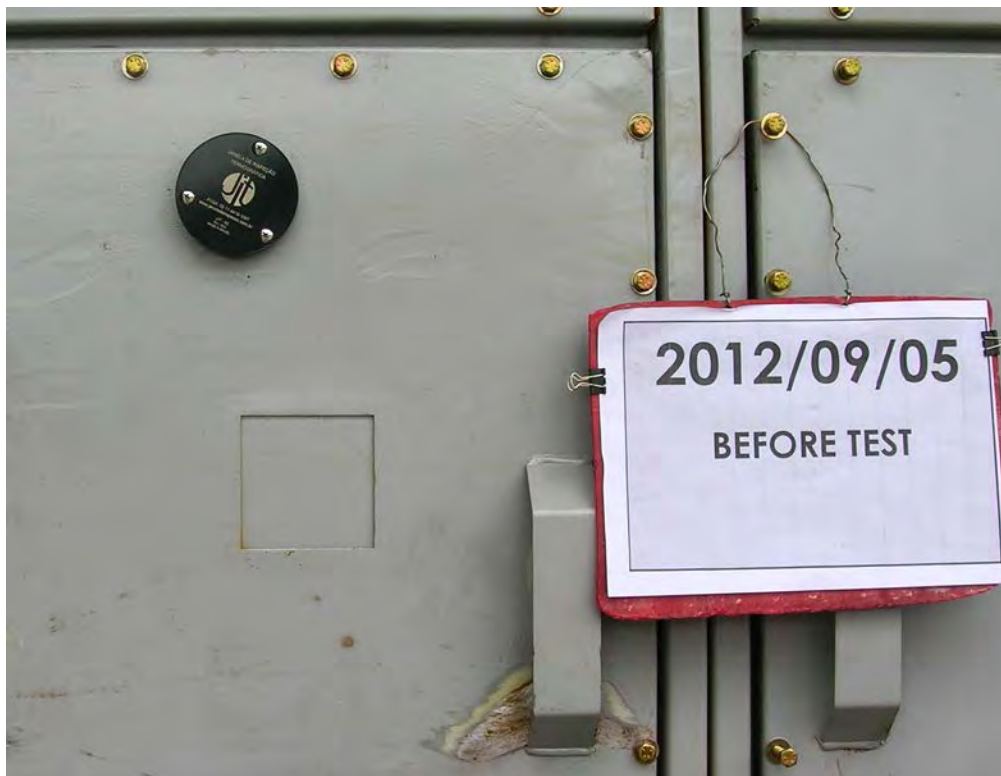
Photo 18 – Before test (InfraPred JIT50)
